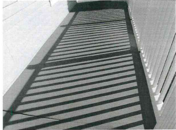
Waterproof coating at concrete breezeway
