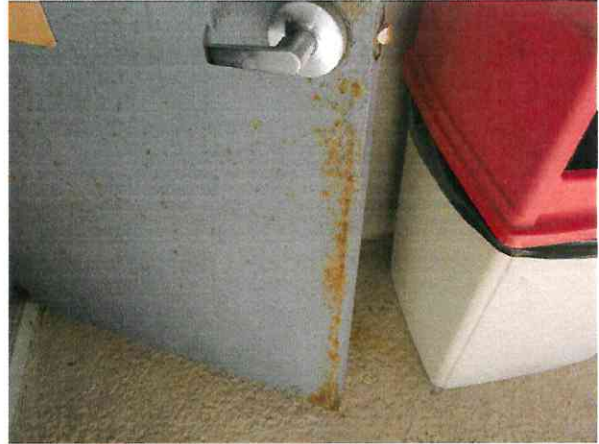
Rust formation at pool mechanical room door
