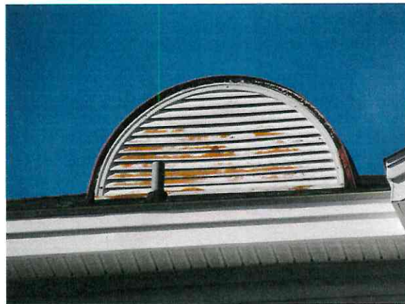
Finish deterioration and rust formation at dormer gable
