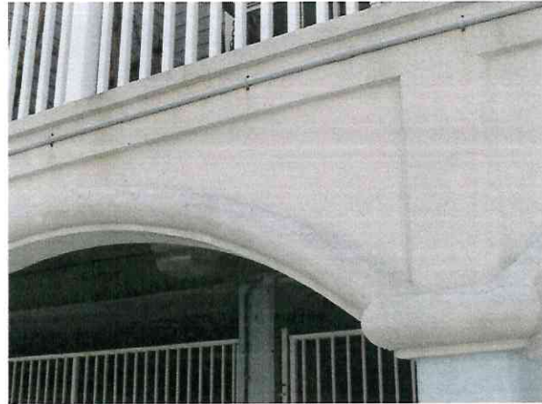
Stains at exterior stucco wall
