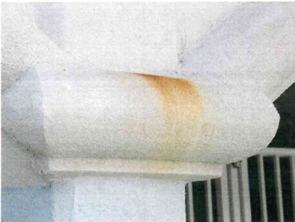
Stain at exterior stucco wall
