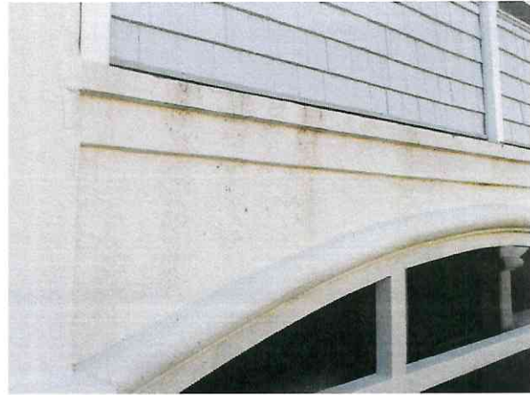
Stains at exterior stucco wall
