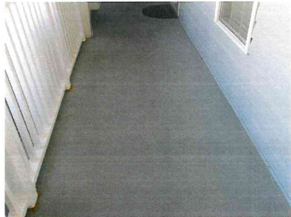
Waterproof coating at concrete breezeway
