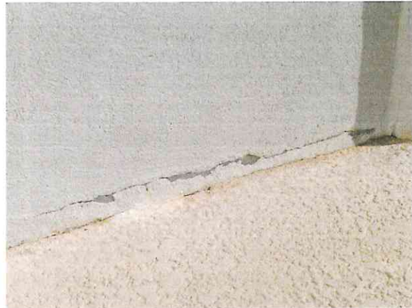
Stucco crack and deterioration at base of exterior wall
