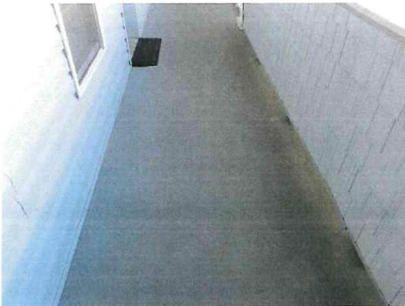
Waterproof coating at concrete breezeway
